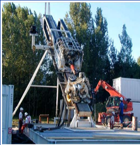
Low Cost drilling
