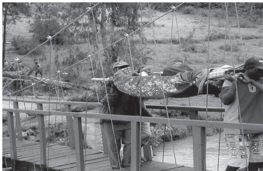
Figure 1. A students' community project in Rwanda built a suspension bridge to cross a 40-metre span of river where a bridge had been washed away, giving the community access to markets and a hospital.
