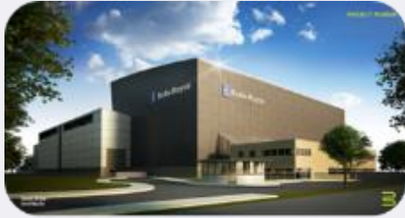
Primary Plant Modules
