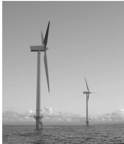
Blyth Offshore, the first offshore wind farm in the UK, with two 2-MW Vestas V66 turbines. Picture:AMEC Wind.
