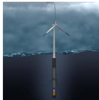
Courtesy - Statoil-Hydro HyWind floating turbine schematic Turbine capacity: 2.3 MW, Height 65m, Rotor diameter: 82.4 m Weight of turbine: 138 tonnes, Total weight: 5300 tonnes Draught below sea surface: 100 m, Sea depth range: 120 - 700 m
